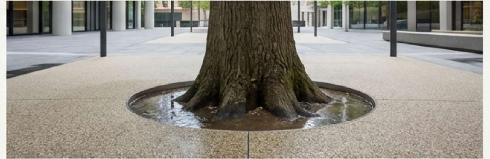
Tree Surrounds: Provide a permeable, stable surface that protects root systems.
